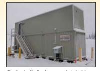
The Alyeska Pipeline Company selected a fully self-contained AdvanTex system with optional control room for a remote site serving pipeline workers in central Alaska. Installed in 2009, the system is producing <5 mg/L BOD/TSS and fecals of <3 cfu/100 mL.
